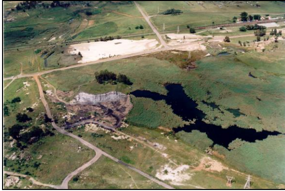
Figure 2. Ponding at West Pit
