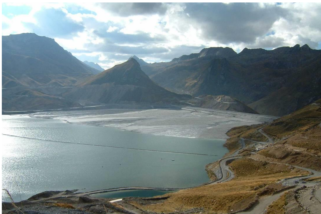
Figure 7. View of Tailings Impoundment from diversion channel showing pond and beach with dam crest. Present Elevation: 4045 m.
