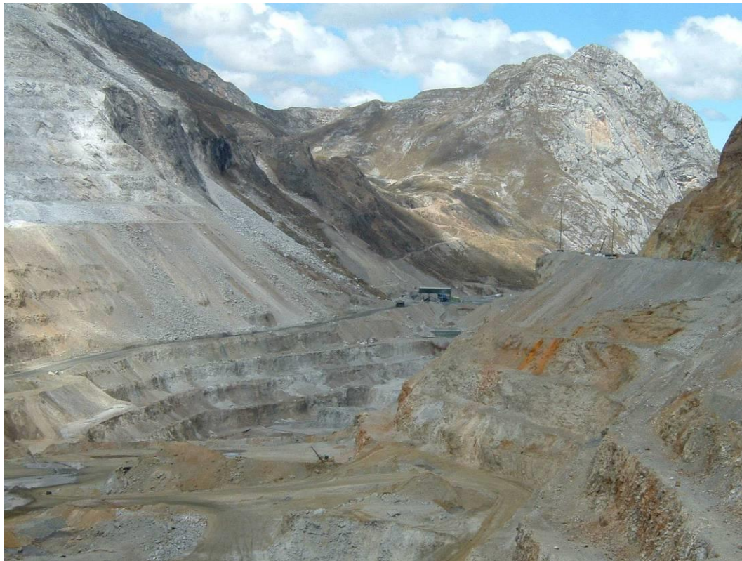
Figure 6. View south of open pit, along Qda Antamina valley. Note in-pit crusher.
