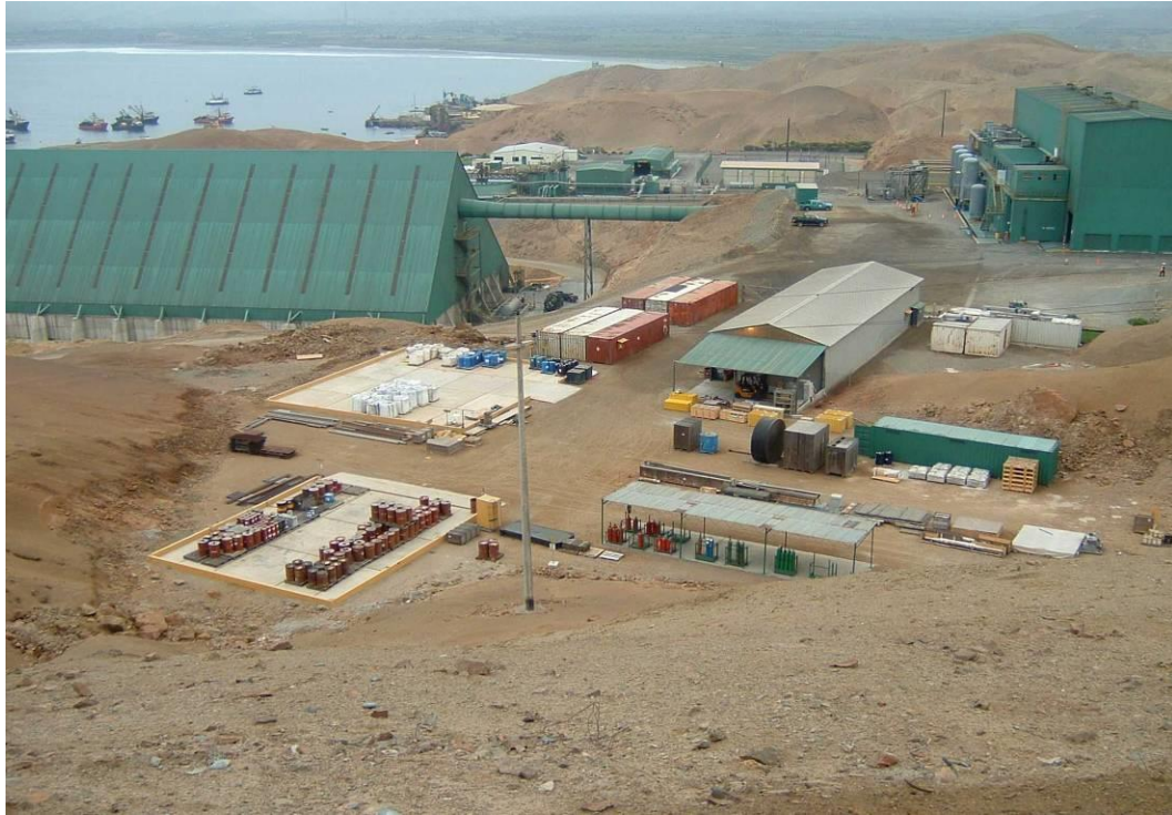
Figure 10. Warehouse and storage area.
