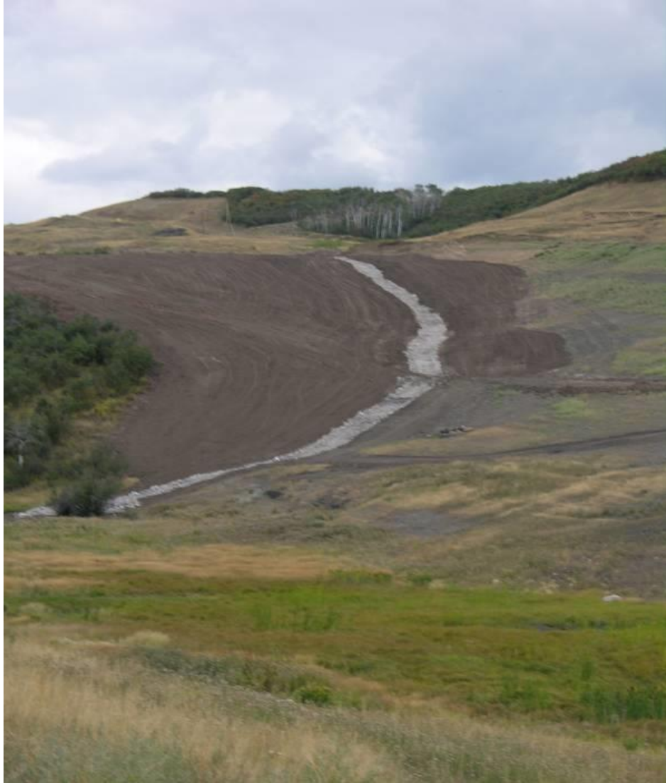
Photo 4. Reconstructed drainage channel and freshly replaced topsoil.
