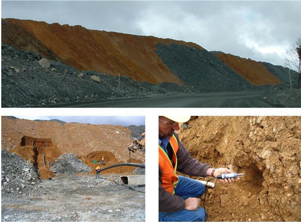
Figure 6 Upper South West Dump Construction and Instrumentation
