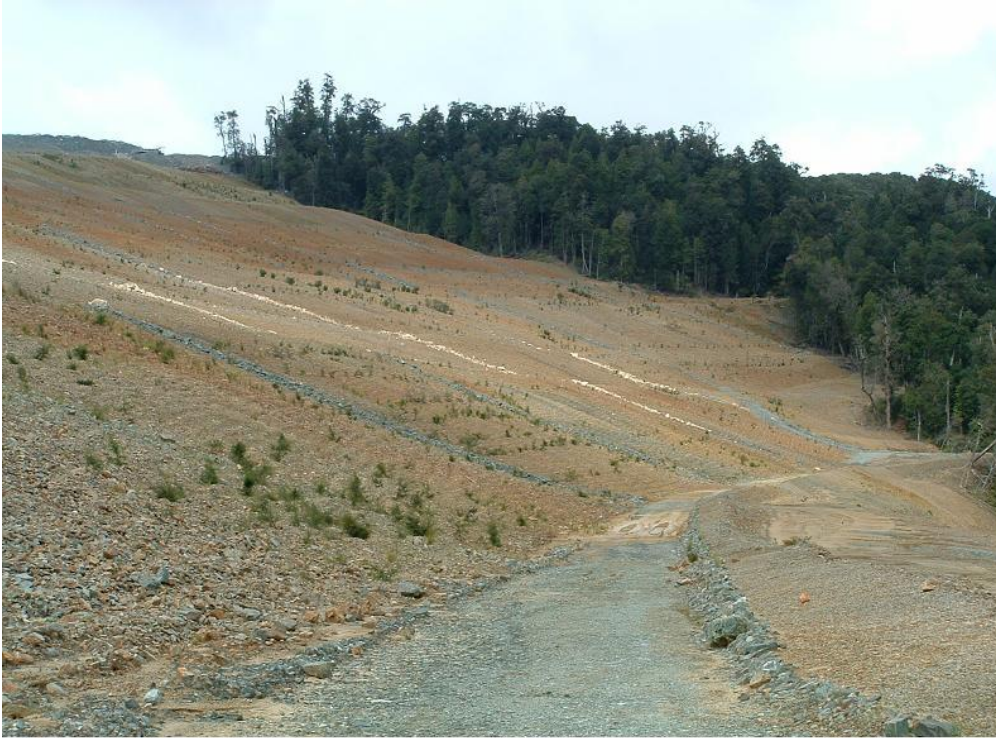
Figure 4 South West Rock Dump – compacted clay encapsulation and re-vegetation
