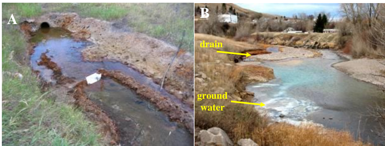
Figure 4. Photographs of the Anaconda Drain. A – View of the Anaconda drainpipe and flume (white) for gaging flow; B – Confluence of Belt Creek (foreground) with the combined AMD from the Anaconda and French Coulee drains (upper arrow). View is looking downstream. The white precipitates in the foreground are hydrous aluminum oxides forming where pH 4.5 groundwater is entering Belt Creek from the left (lower arrow). [Photo by C. J. Fisk, Nov., 2005].
