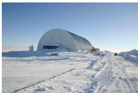
Figure 2. Exterior of Raglan plant
