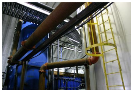
Figure 3. Interior of Raglan plant
