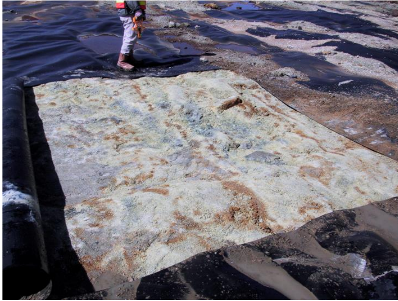
Figure 11. Oxidation products discovered underneath the HDPE geomembrane cover during decommissioning of the trial dump.
