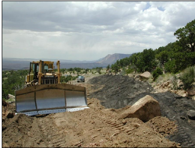
Figure 13: Reclamation of the main mine access road utilizing existing soil material.
