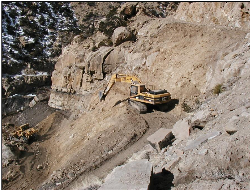
Figure 7: Substitute soil excavation between the switchback area of the upper mine
