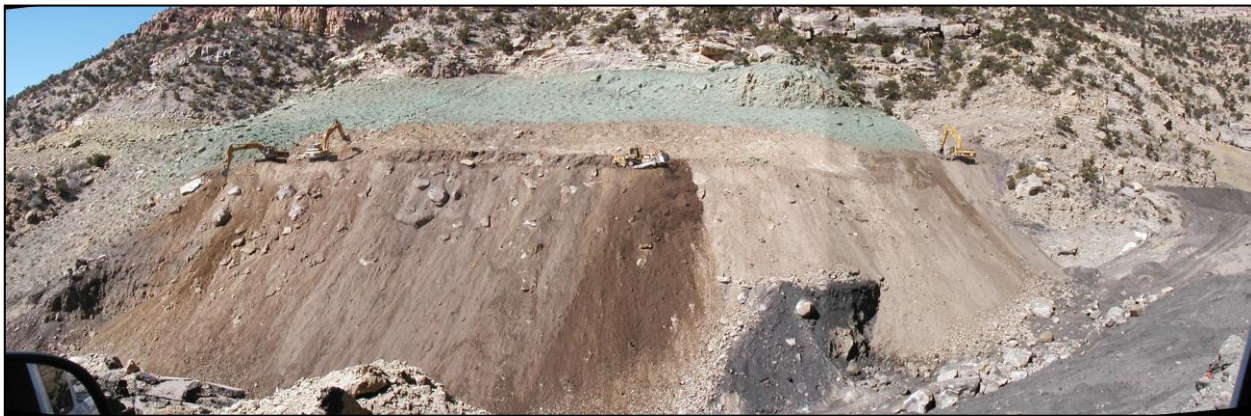
Figure 12: Re-working the bathhouse slope. Equipment traverses back and forth casting material to bottom of canyon.
