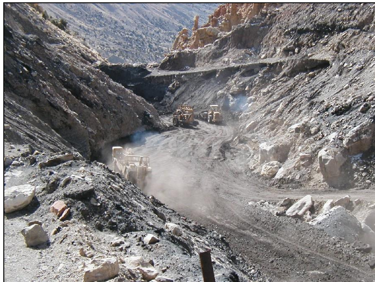
Figure 9: Placement and compaction of spoil material in canyon bottom.
