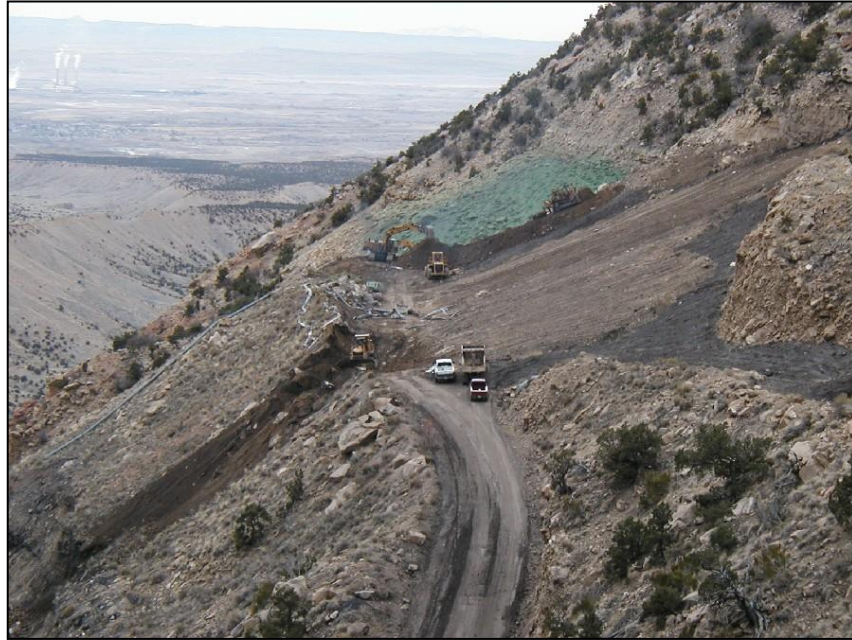
Figure 11: Covering bathhouse fill slope with topsoil.
