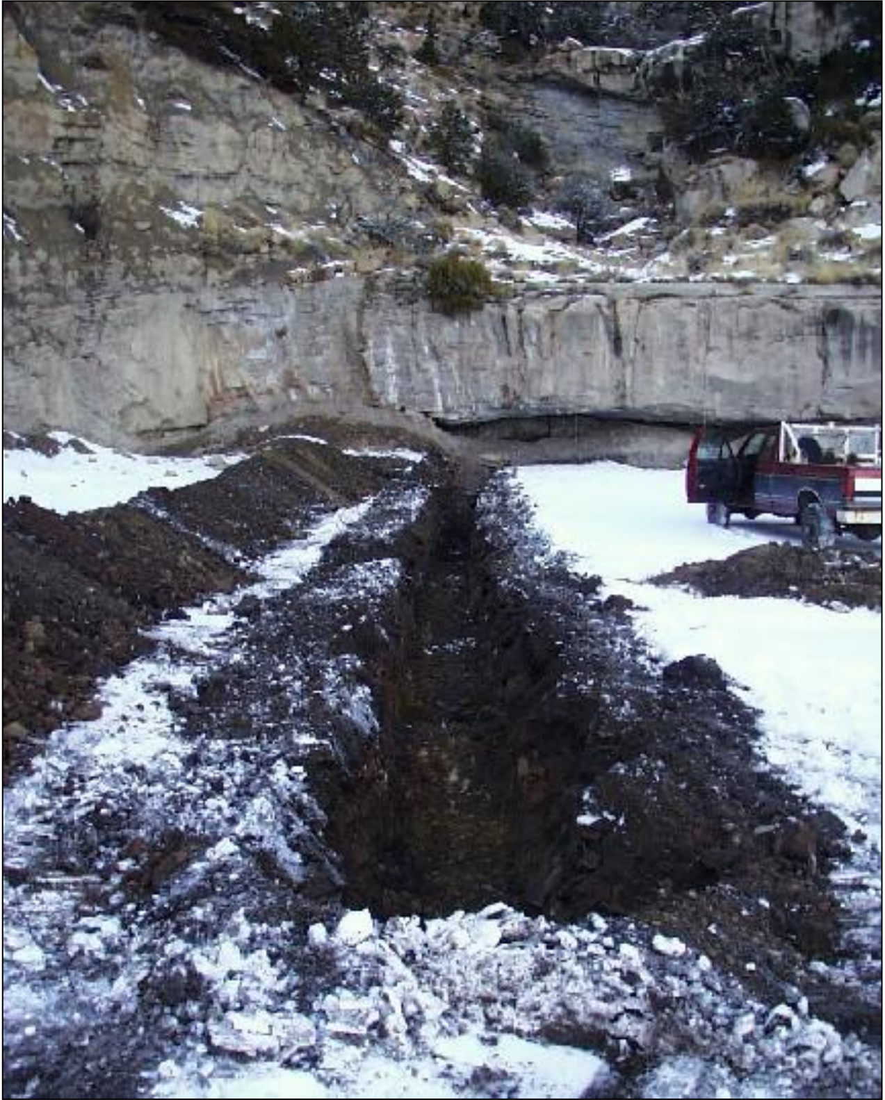
Figure 3: Trench #2 developed on the upper mine pad.
