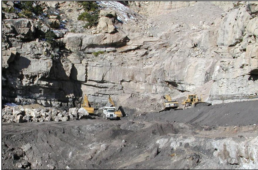
Figure 6: Backfilling highwall with spoil material at the lower mine portal pad.
