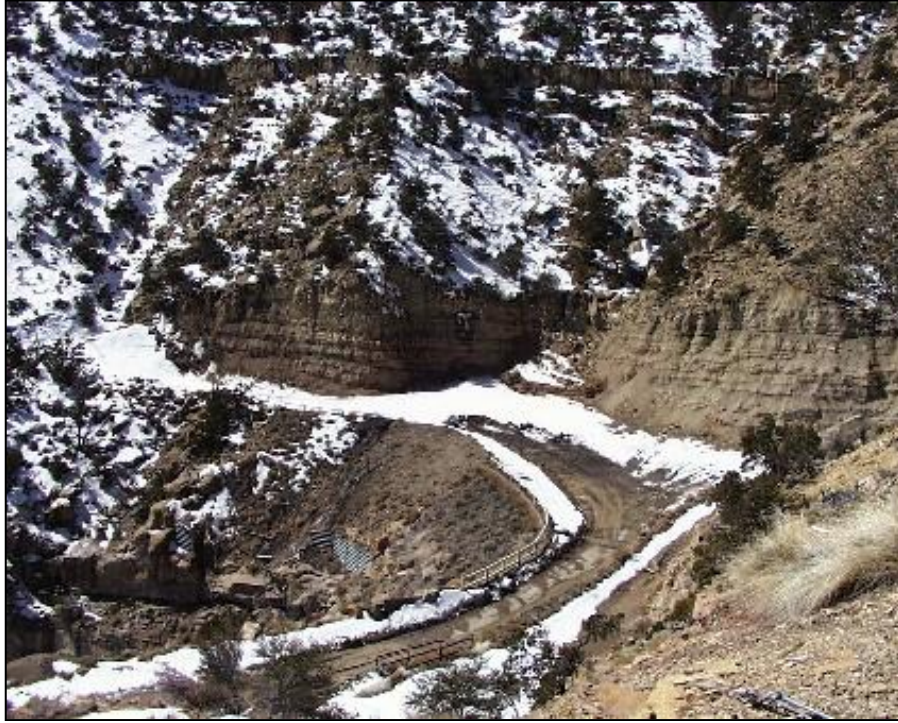
Figure 4: Upper mine portal of the Phase 1 area prior to backfilling and grading activities.
