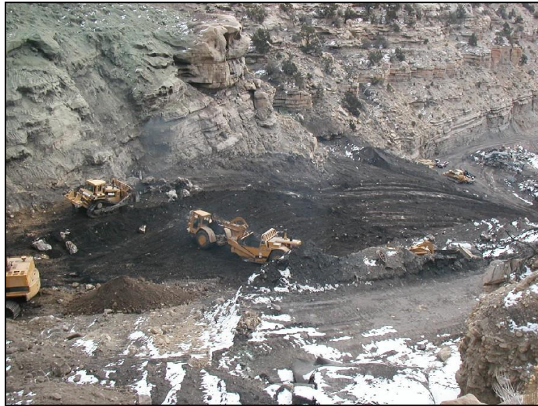
Figure 8: Removing spoil material by dozer and transporting with scraper down canyon.
