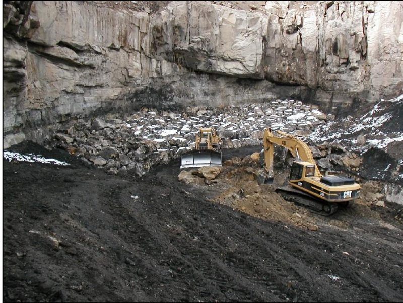
Figure 10: Commencing excavation of the upper channel to uncover the bedrock contacts.
