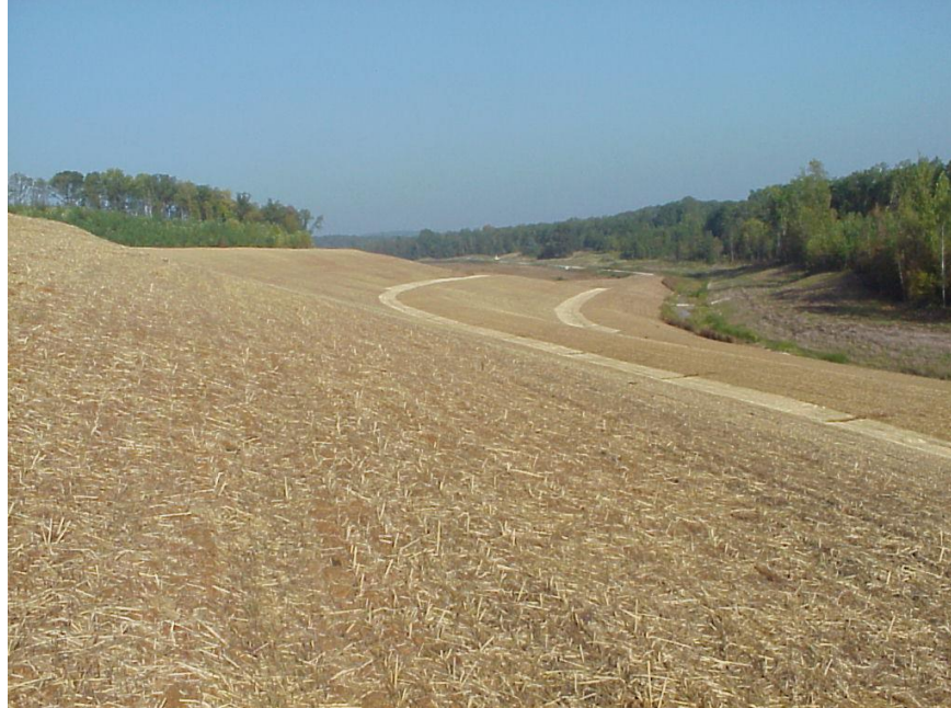
Figure 3. Seeded and mulched upland area with erosion fabric lined water bars.
