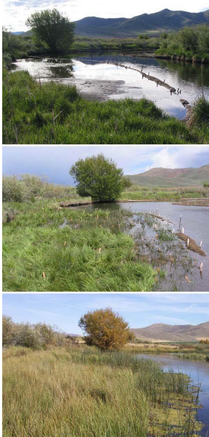
Figure 4. Pre-planted coir was used to revegetate filled areas in this project that narrowed an over-widened spring creek in south-central Idaho. Individual transplants had failed previously. From top to bottom: before installation, immediately after installation at the beginning of June, 2005, and in September, 2005.
