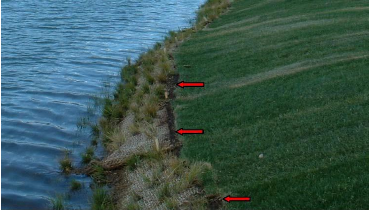
Figure 10. Slumping of pre-planted coir blankets on this pond shoreline resulted from fluctuating water levels and insufficient depth of fill over a synthetic liner. Slumping exposed the band of soil indicated by the arrows. Poor growth and drying of plants also reflects the inadequate soil depth, which was less than specified in the design. Fill and vegetation both had to be replaced.
