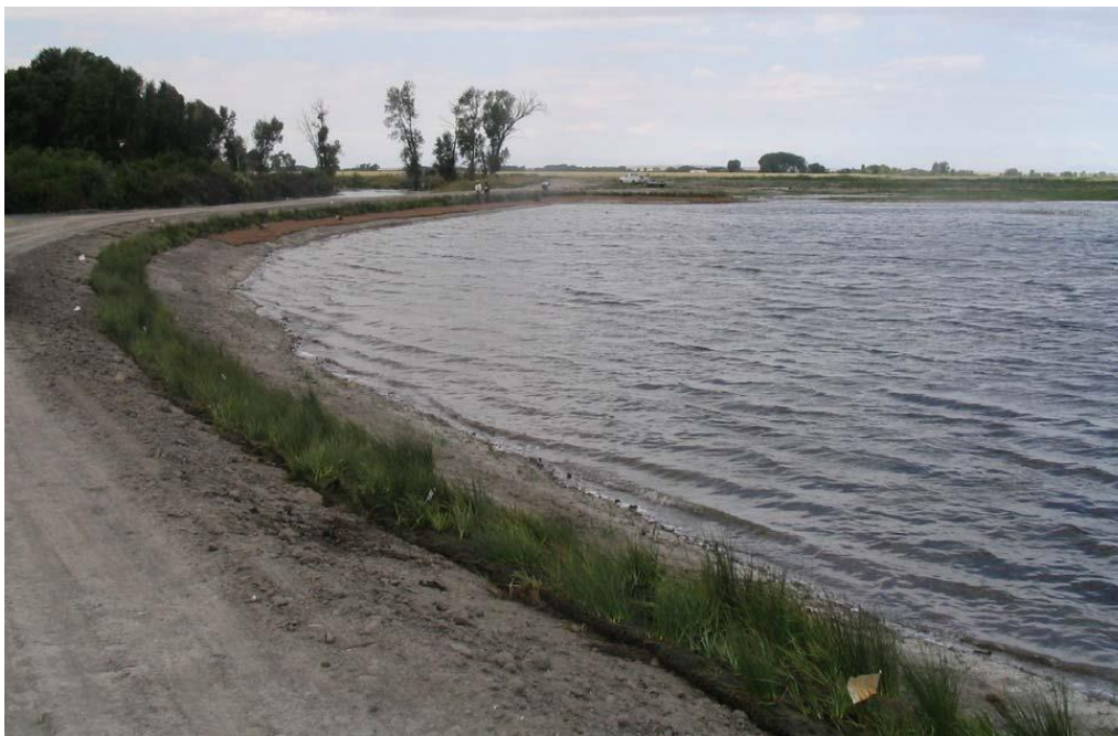
Figure 5. Pre-planted coir blankets installed at this site required temporary irrigation because target water levels (level of vegetation in photograph) were not reached on schedule. Water for the pond was supplied by a large irrigation canal that had more than adequate capacity to fill the pond on time, but withdrawals by upstream irrigators during warm weather delayed filling more than anticipated.
