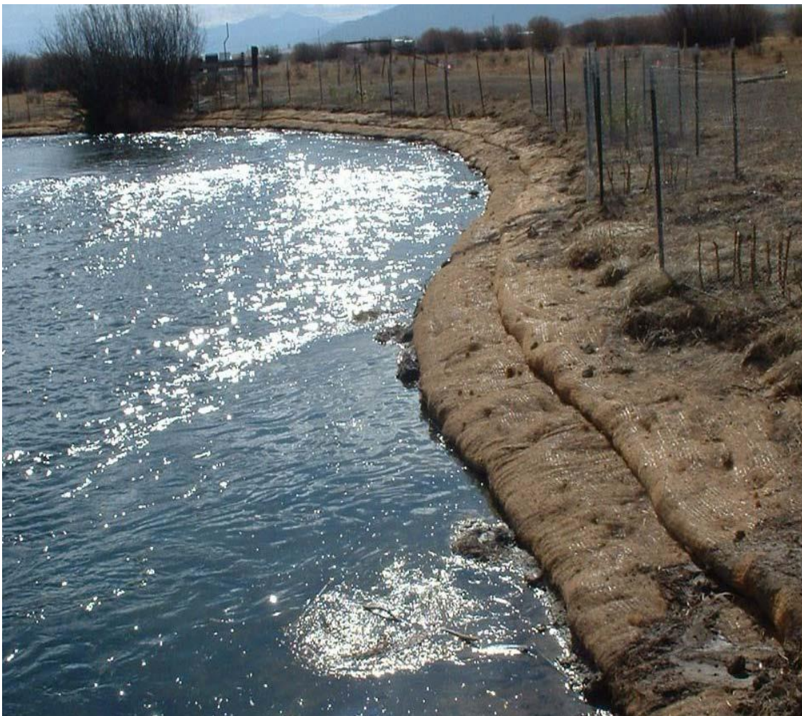
Figure 11. This bend in the Teton River, Idaho, was rebuilt with a gentler slope and protected with erosion control fabric before installing pre-planted coir blankets. Two lifts of soil are protected by separate pieces of ECF, each with its lower edge buried before folding it back over the soil “burrito-wrap style”. Fencing protects young shrubs on bank from browsing.
