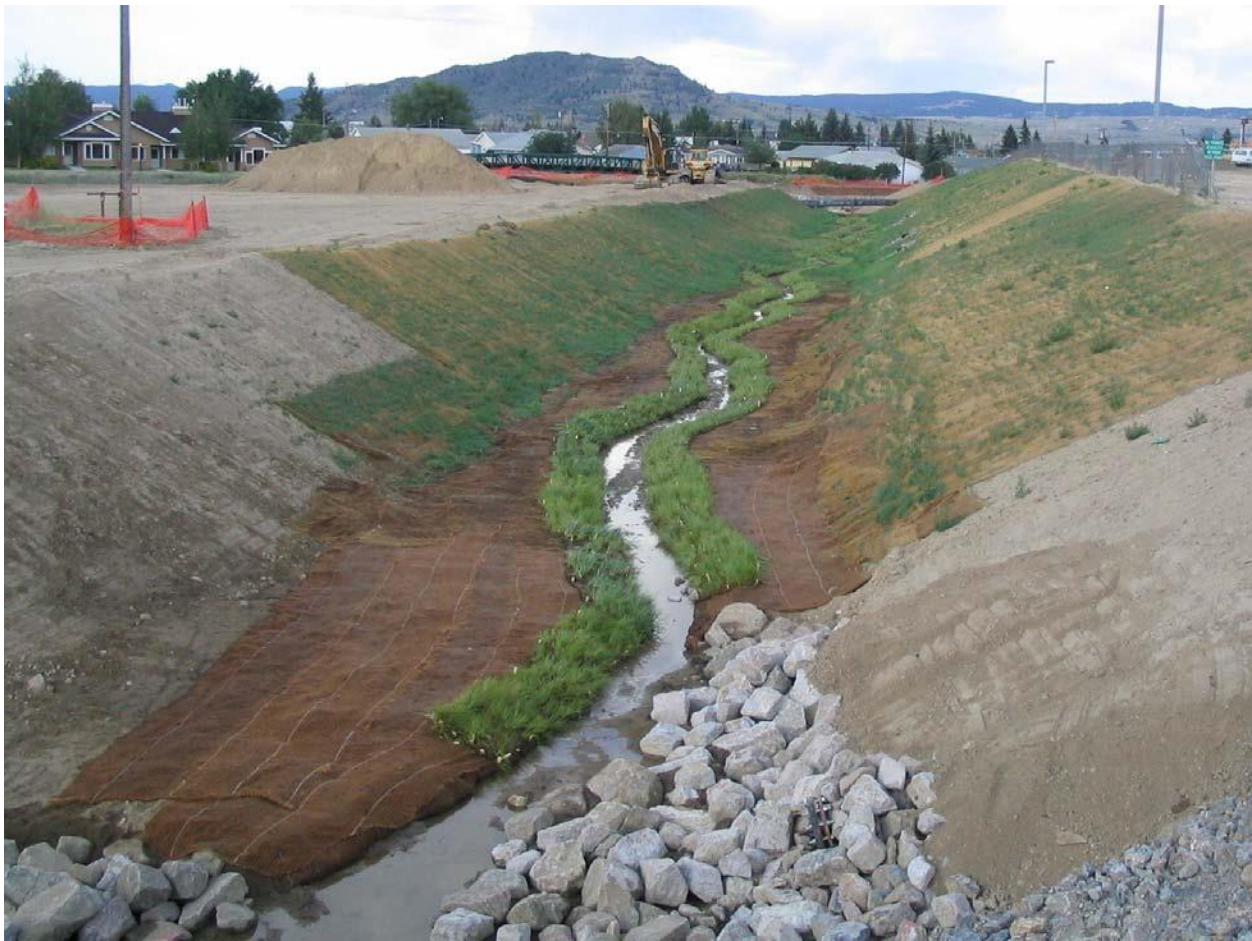
Figure 12. In the Butte Metro Storm Drain Reconstruction project, pre-vegetated coir blankets were a small but important feature of a complete design. The form and size of the large trapezoidal channel used standard hydrologic analyses and engineering methods to design for flashy urban runoff, and the entire bottom of the channel was armored with coarse aggregate before placing topsoil. The small, sinuous pilot channel in the center is designed largely for aesthetics and carries a low, seasonal base flow. Pre-planted coir was used on the banks of this pilot channel in many areas, but other materials such as rock revetments were also used. Erosion control fabric was installed over all top-soiled areas. Areas away from the channel banks were seeded, and woody species were planted on upper side-slopes. This channel handled a large runoff event successfully just 10 days after pre-planted coir was installed (Hook 2006).
