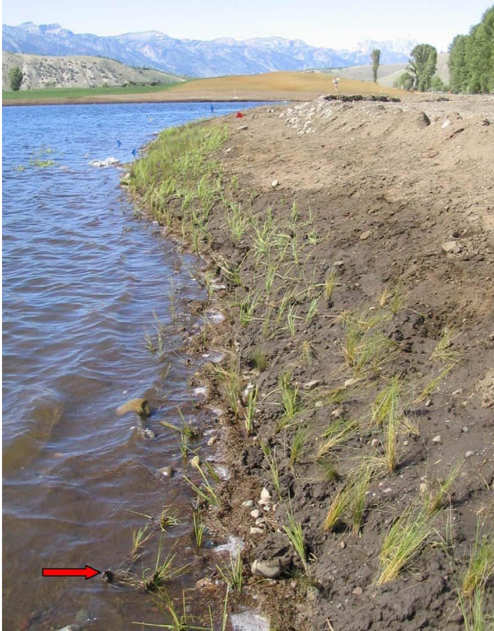
Figure 9. Even gentle wave action can be destructive on unprotected shorelines. On this shoreline, topsoil was placed over an artificial liner and planted with individual tubelings. When this photograph was taken, minimal waves caused by moderate winds had started to erode soil and dislodge plants at the waterline (e.g. at arrow). Other shoreline areas at the same site that were protected with pre-planted coir tolerated larger waves.
