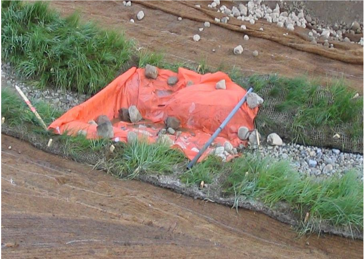
Figure 14. Temporary tarp dam used to raise upstream water levels to irrigate newly installed pre-planted coir blankets in the Butte Metro Storm Drain. A pipe or pole supports one edge of the tarp across the channel, and rocks are used to hold the tarp against the channel bottom and sides. At this site, base flow is artificially controlled but limited. The photograph was taken when the channel was drained to allow dams to be moved.
