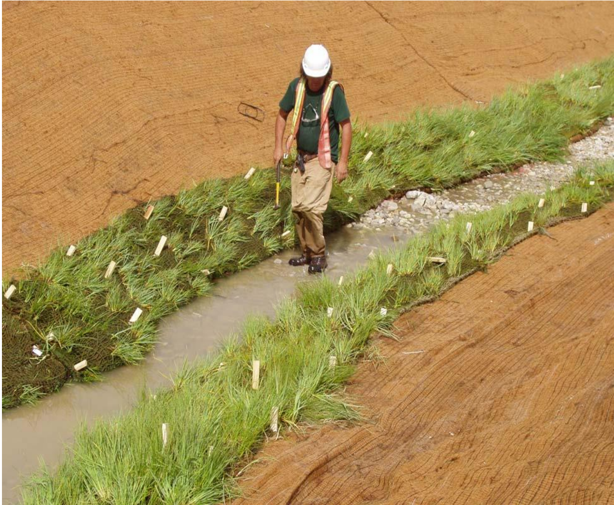
Figure 13. In the Butte Metro Storm Drain Reconstruction project, pre-planted coir blankets were staked at relative high density, with stakes angled to help secure the coir against currents.
