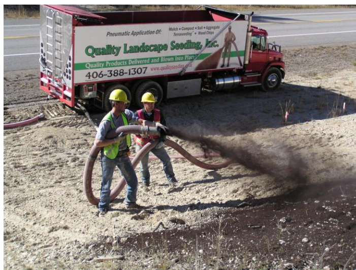
Figure 12. Express Blower Model EB-30 applying compost at the Middle Thompson Lake site.
