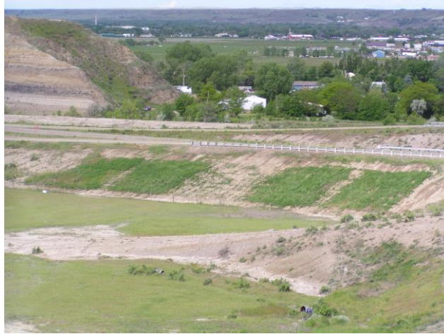
Figure 19. Mile's City I-94 Off Ramp Plots, Spring 2005
