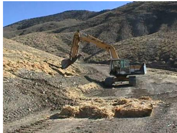
South Waste Rock Dump Plant Growth Medium, Mulch, and Ripped Surface under construction
