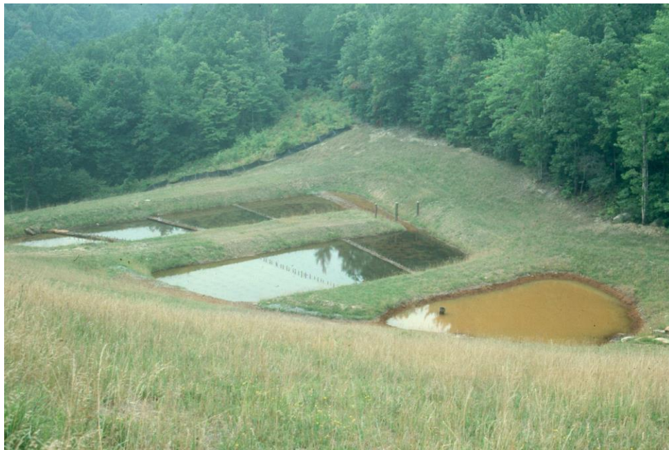
Figure 4. The WV-34 site contains six cells, the first three are seen here. The first red pond collects the seepage from the hillside, then the water is routed through these anaerobic cells. This system has removed an average of 39 g/m 2 /day.
