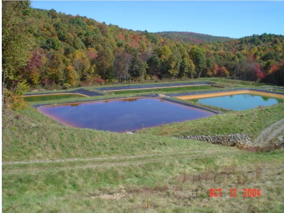
Figure 6. The WV-15 VFW and Pond systems received acidic water (in the foreground) from seepage, which was routed through the WV-15c VFW, then to the WV-15a Pond. From there, the water flowed through the WV-15d VFW and then through the WV-15b Pond. The 15-c VFW removed around 7 \text{ g/m}^2/\text{day} , the 15-d VFW removed around 2 \text{ g/m}^2/\text{day} , while the Ponds removed only small amounts of acidity ( <1 \text{ g/m}^2/\text{day} ).
