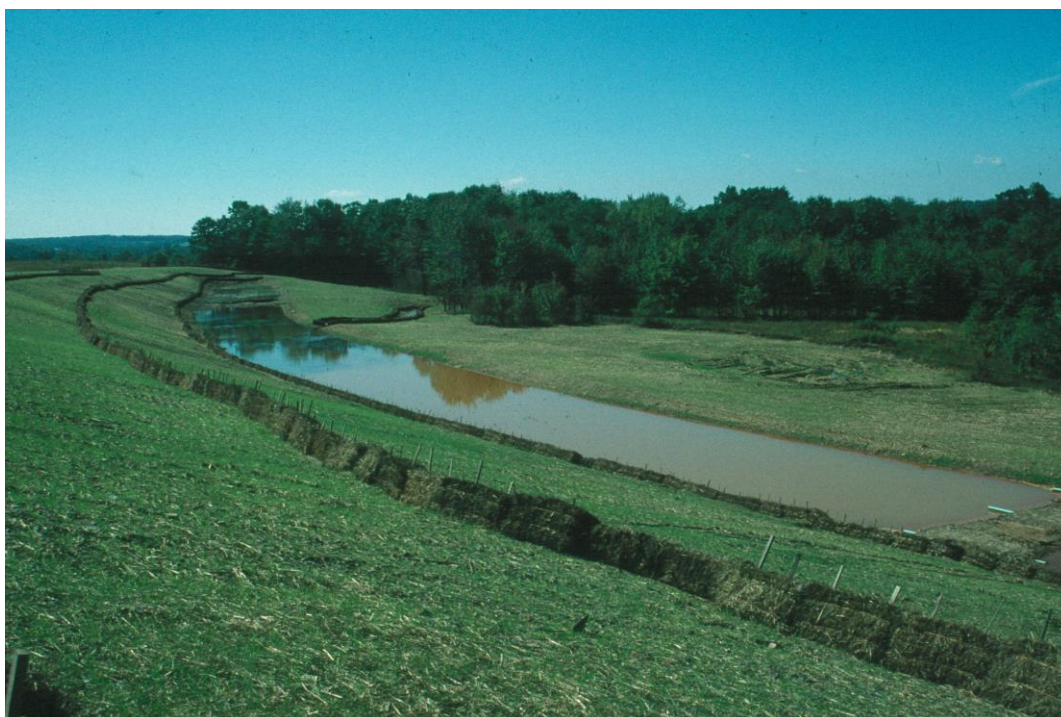
Figure 2. The WV-4b anaerobic wetland systems (AnW). This wetland system removed 3.9 g/m 2 /day.
