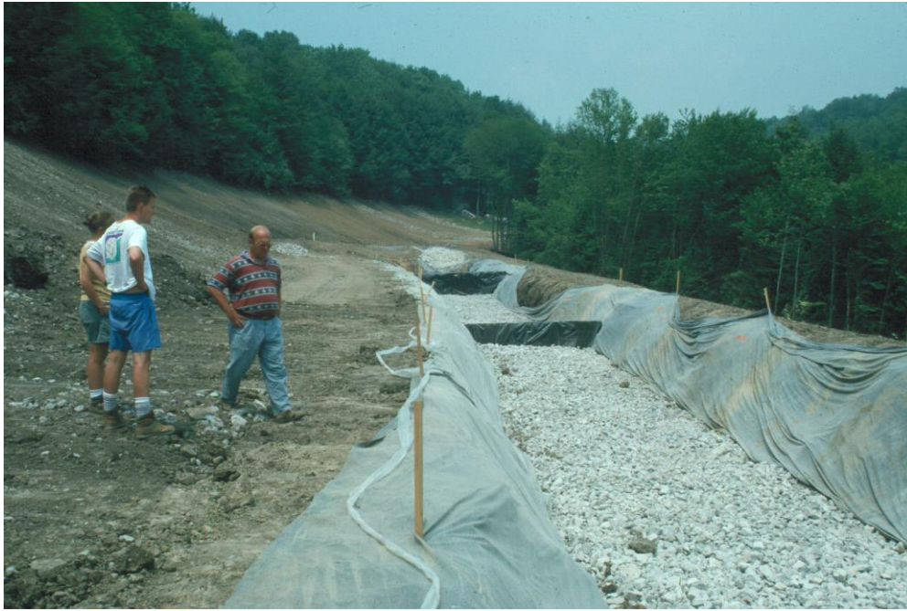
Figure 5. The WV-1a ALD removed an average of 74 g/day/t of acidity, which was a high removal efficiency for ALDs.
