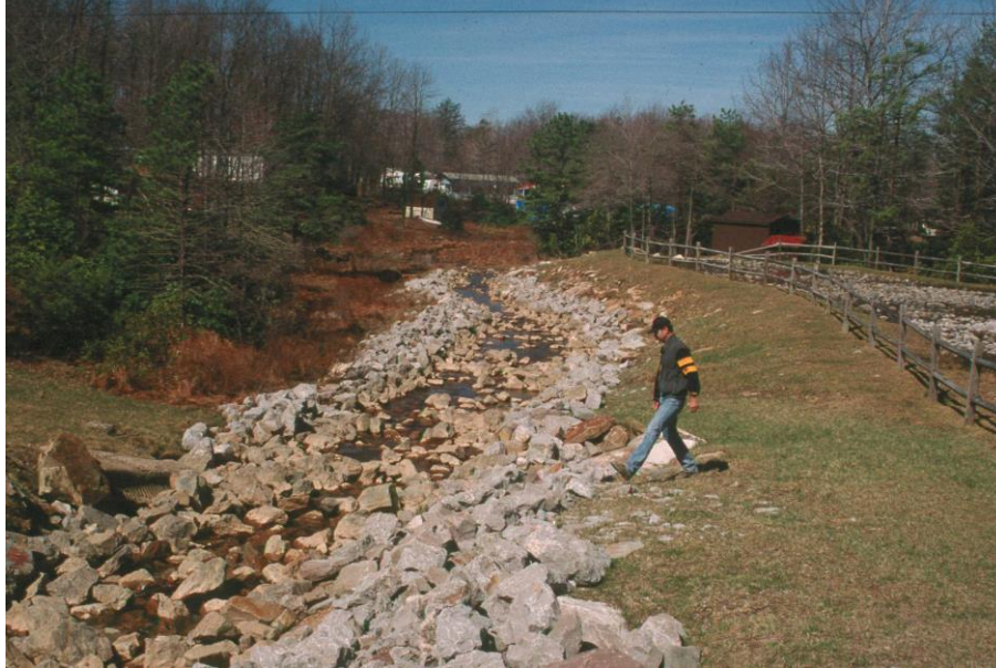
Figure 7. The WV-36a OLC had the highest removal efficiency of all the OLCs we sampled at 121 g/day/t. The influent water had a pH of about 5.5 with no metals.
