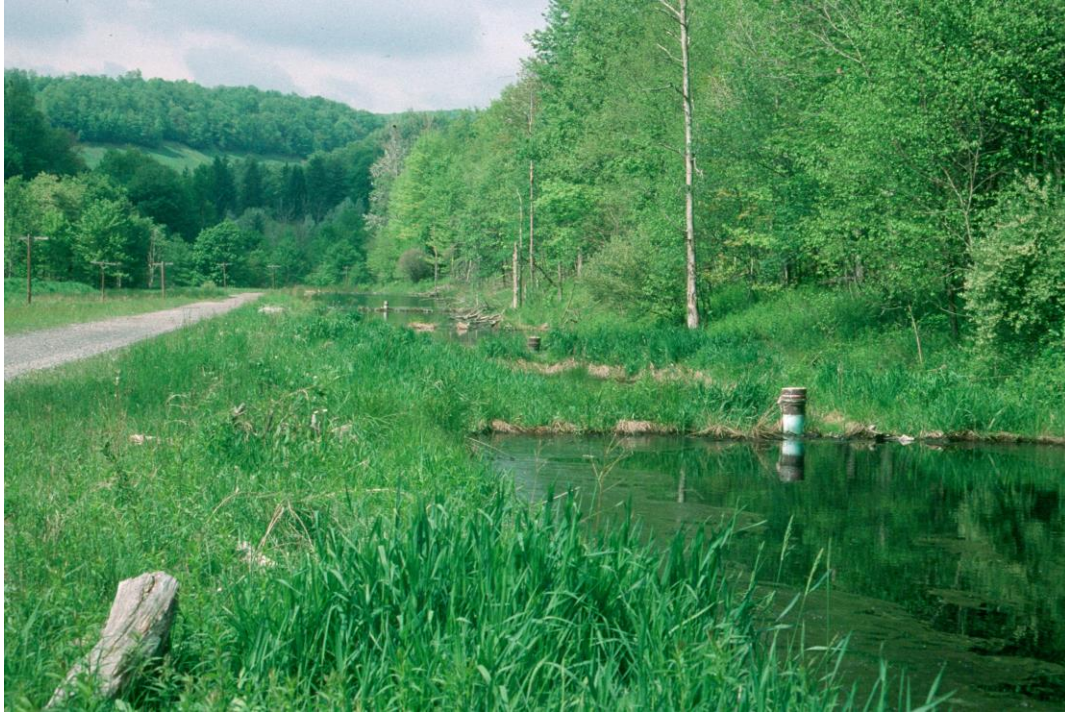
Figure 3. The WV-6 AnW system is a long narrow wetland along an abandoned railroad. The system was expensive to build but removes 33 \text{ g/m}^2/\text{day} .
