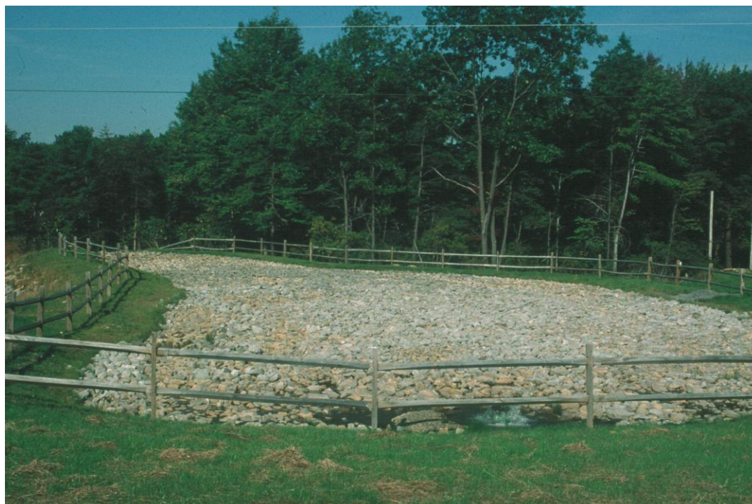
Figure 9. The WV-36d LSB receives low pH water with no metals. Under this condition, the limestone is not armored and continues to dissolve. The removal efficiencies have remained constant from 10 g/day/t in 1999-2000 to 14 g/day/t in 2004.
