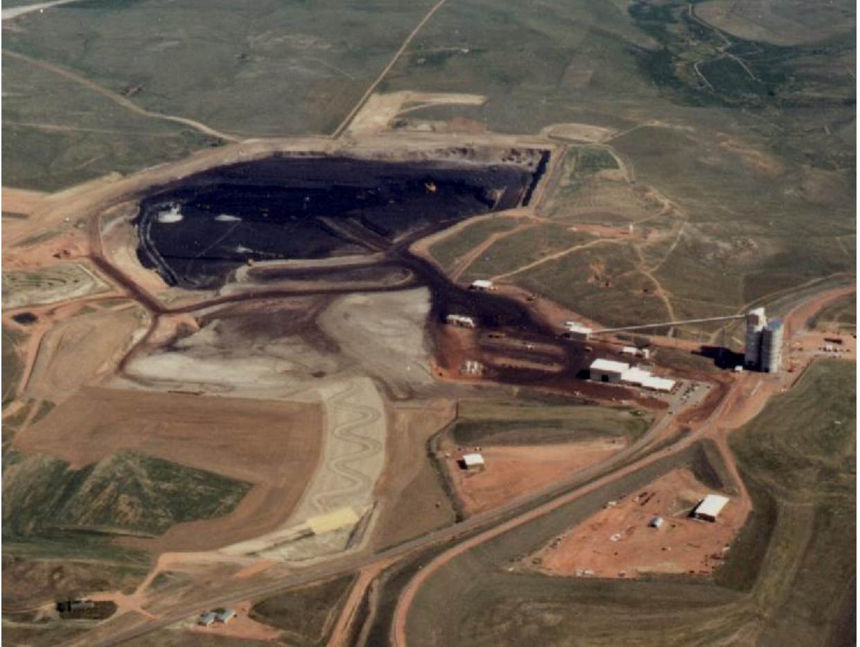
Figure 6: Caballo pit in June 1981. Photo is looking north. (Area A wells are located where backfilling is taking place north of meandering reclaimed North Tisdale Creek). Native North Tisdale Creek trends to northwest in photo.
