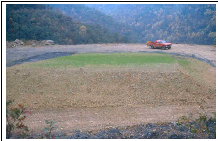
Figure 3. View of recently constructed and seeded topsoil wedge at Jewell Smokeless Coal (JSR) in 1983. This view is from the rear (high side) of the wedge, looking down from 1.8 m to 0 cm in front of red pickup.
