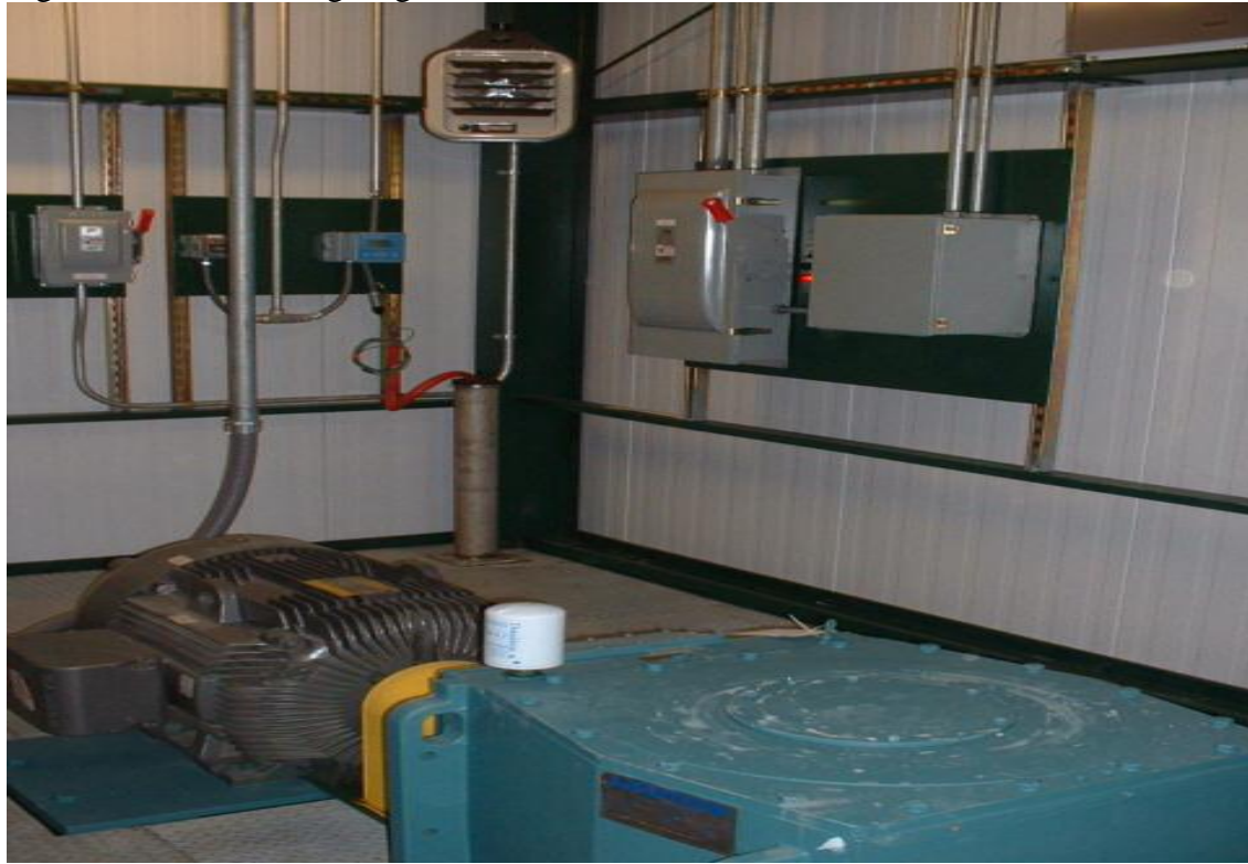
Figure 10. Second Stage Agitator/Aerator Drive Mechanism
