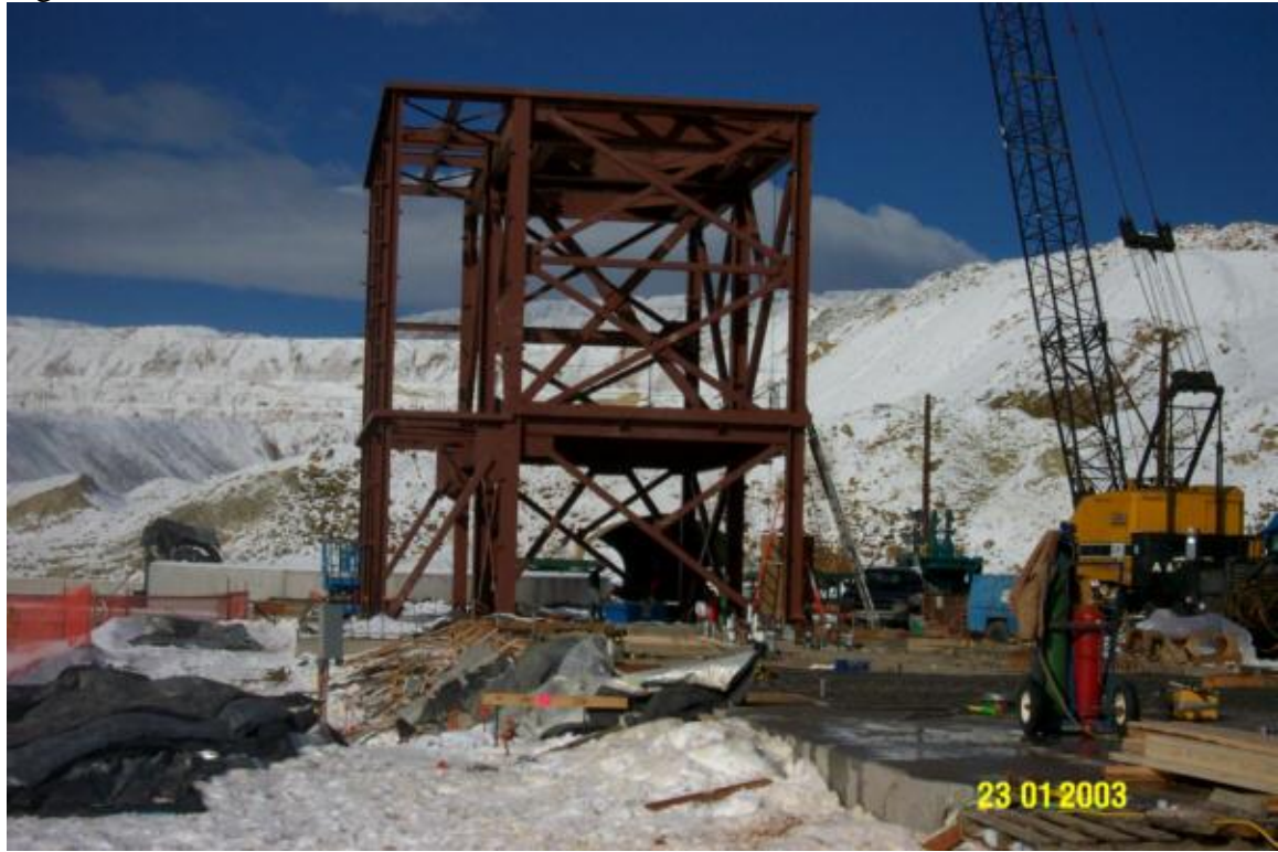
Figure 5. Lime Silo Pre-lift
