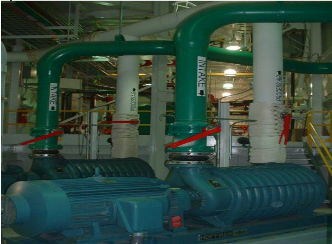
Figure 12. Blower Installation
