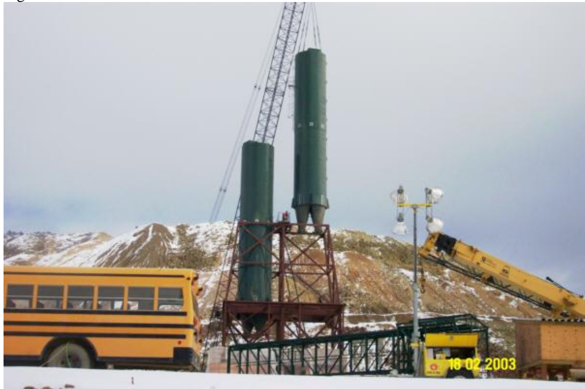
Figure 6. Lime Silo Lift
