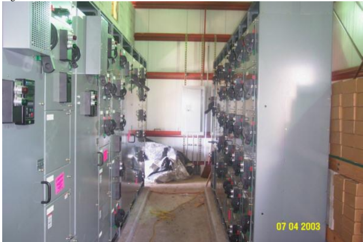
Figure 16. Motor Control Center
