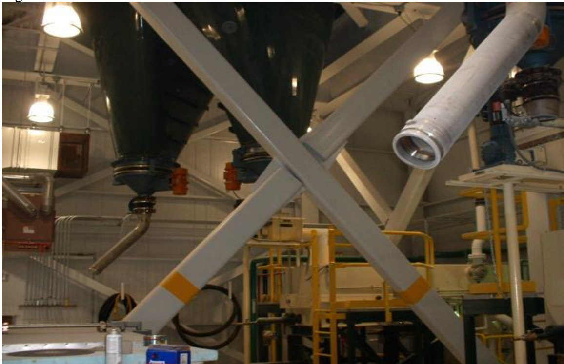
Figure 13. Limo Silo Cones and Slaker
