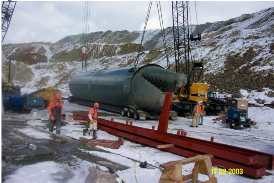
Figure 5. Lime Silo Pre-lift
