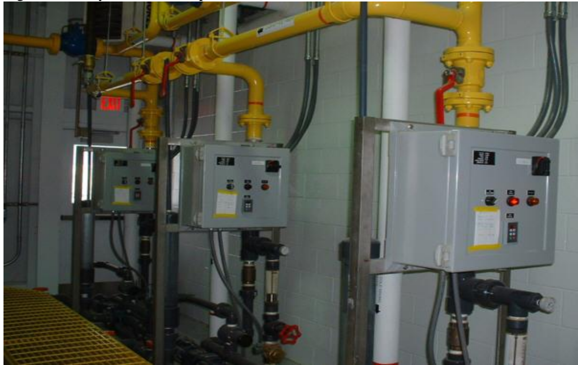
Figure 17. Polymer Feed Pumps and Controls
