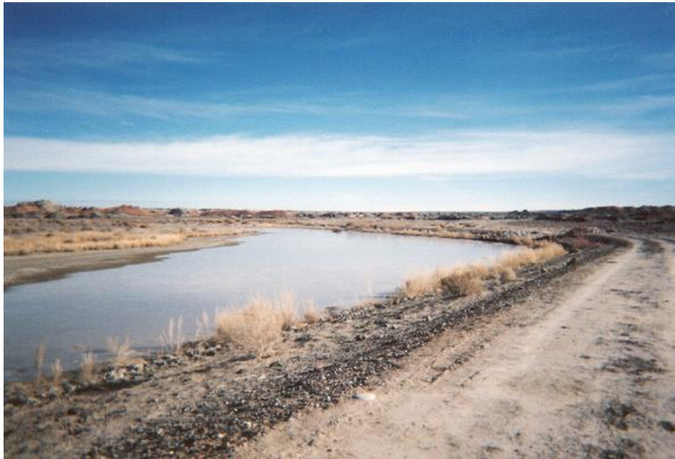
Figure 4. Sedimentation pond and dam at the Gateway Mine. This dam was breached for Phase III bond release.
