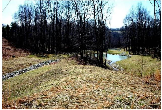
Fig. 6. Limestone and steel slag dam on Beaver Creek of Little Sandy Creek.
