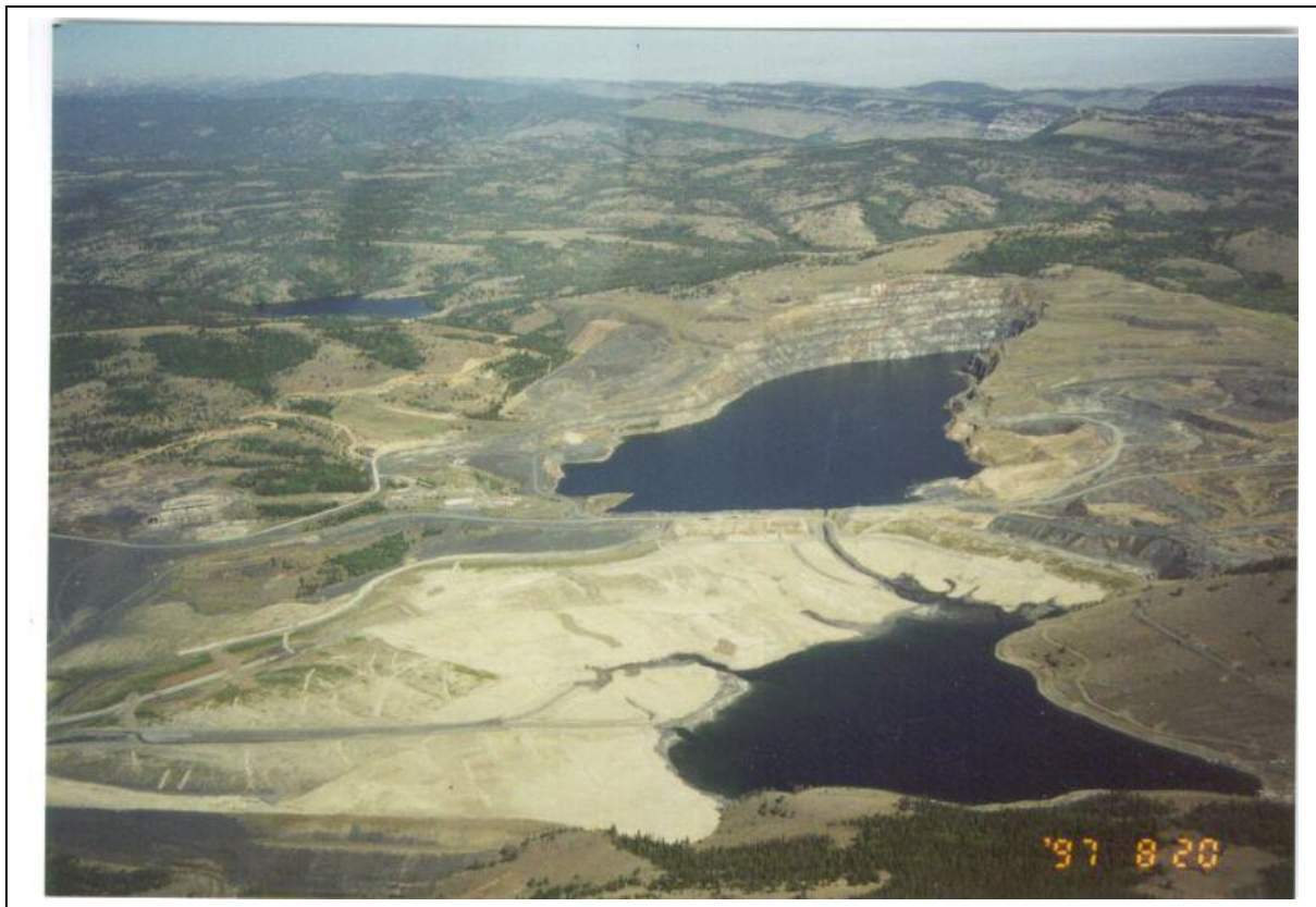
Figure 1 - Atlantic City Iron Mine During Tailings Impoundment Reclamation. Tailings Impoundment In Foreground, Mine Pit In Center, Waste Rock Dumps To Right and Left Of Pit, Plant And Shop Areas At Left Center Above Tailings.
