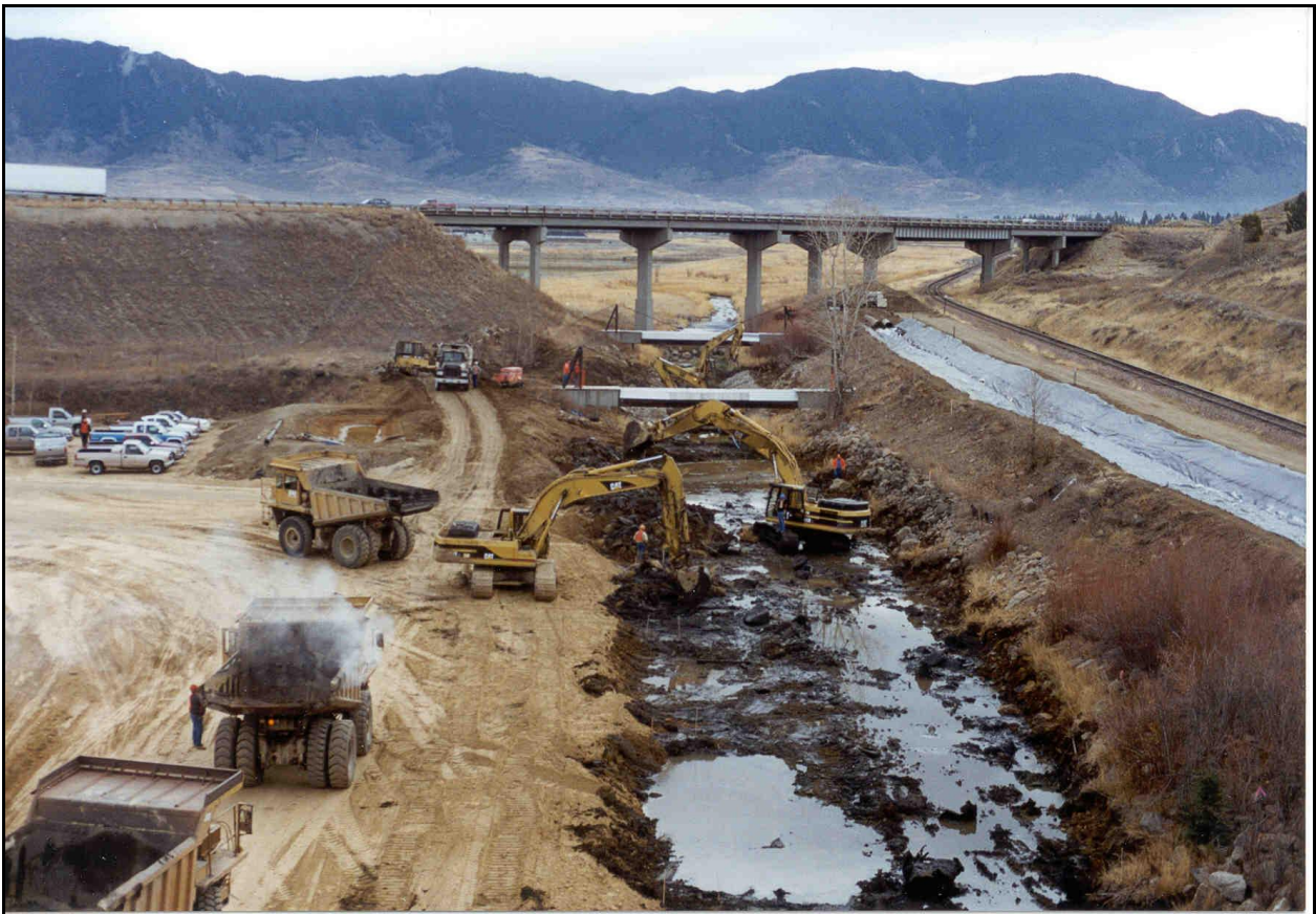
Photo 4. Non-deformable channel excavation with flow in diversion channel at right.
