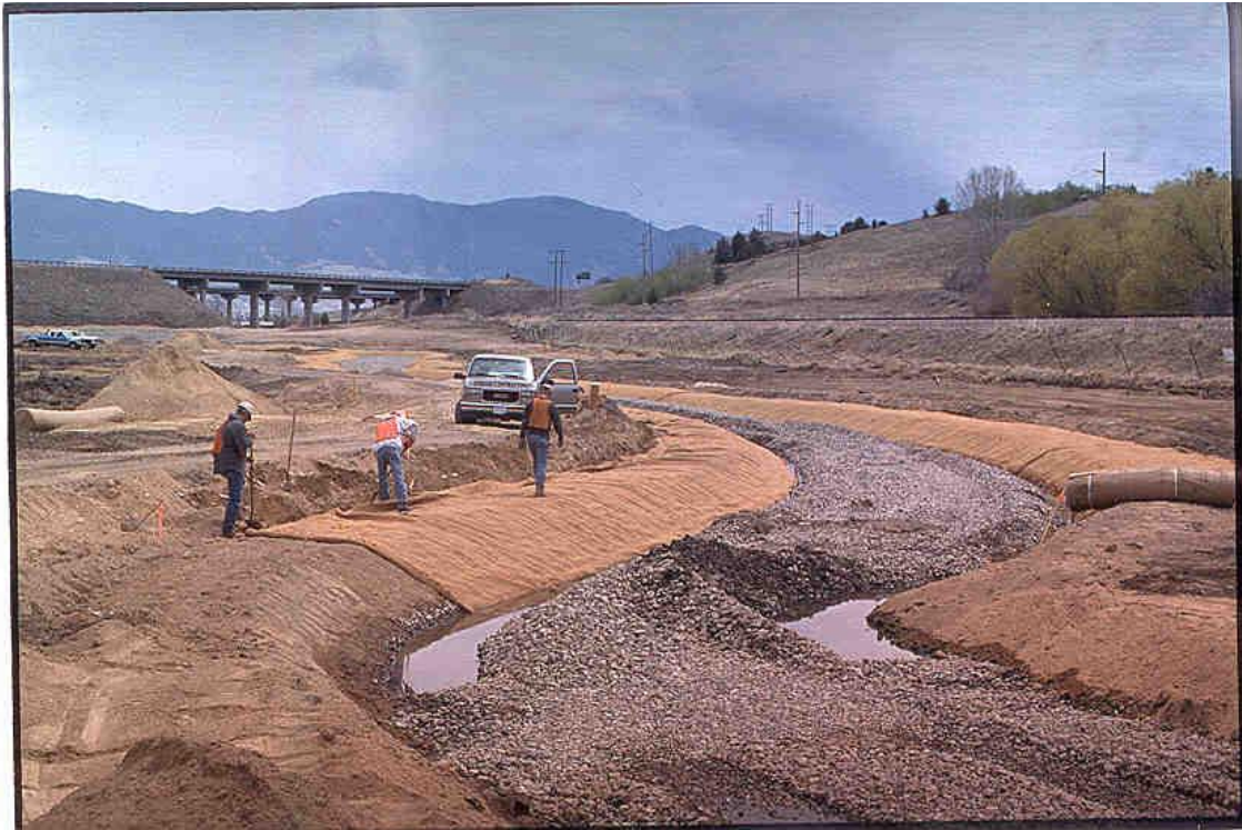
Photo 6. Deformable channel during construction.
