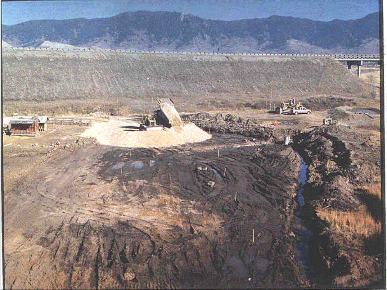
Photo 3. Borrow material being placed over floodplain within SST Operable Unit.
