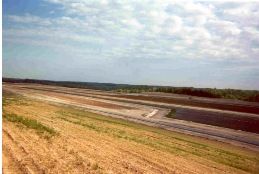
Figure 11. Overview of Stafford Regional Airport in June, 2002. The vegetated area in the foreground was incorporated and seeded by mid-April. The barren area in the background was not completed until late May.
