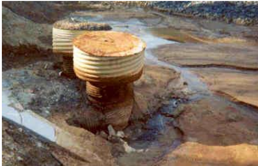
Figure 5. Galvanized steel standpipes in water control structures in storm-water basins below the site have been completely degraded by acidic drainage.
