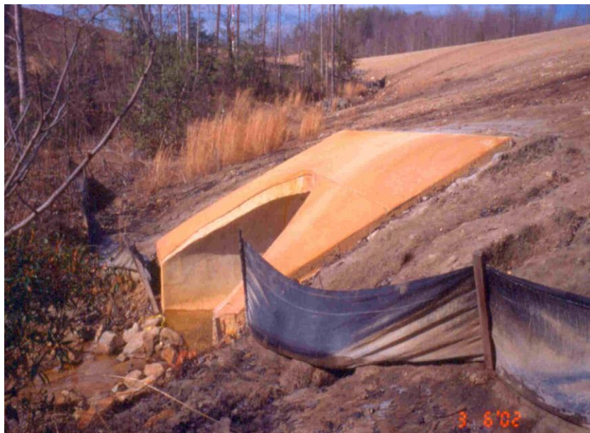
Figure 4. Throughout Stafford Regional Airport, concrete structures such as this culvert exhibit iron-staining as well as etching and degradation of cement components.
