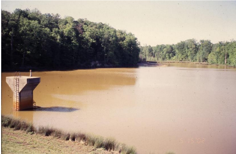
Figure 7. Drainage from Stafford Regional Airport flows off-site to this storm-water basin.
