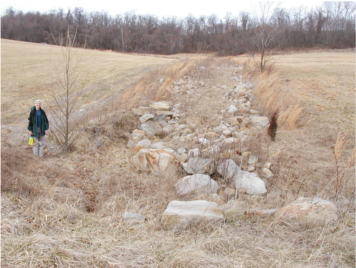
Figure 12. Typical over-sized armored constructed channel. Located at study site 80-80., channel is lined with large sandstone boulders. Approximate bankfull dimensions are 0.5 m deep, 1.4 m wide across the channel bed and 2.6 m wide at top of channel. J.S. Kite photo.
