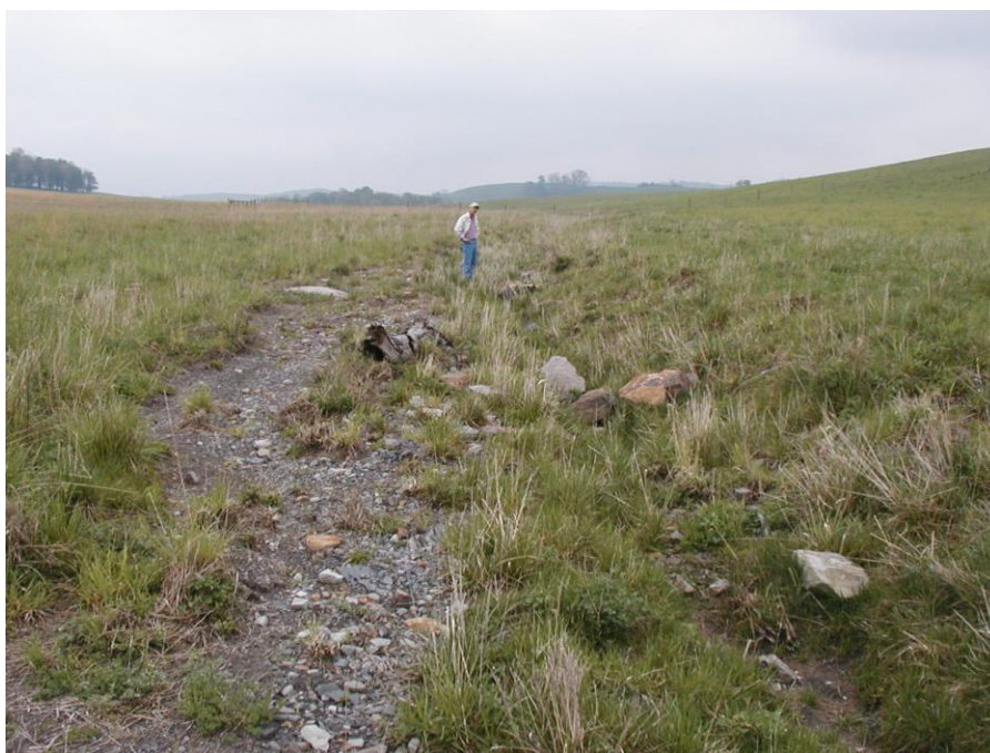
Figure 14. Channel at site 1008-95 downstream from correctly sized channel. Flow direction is away from the camera. Moderate flows have exceeded capacity of channel, scouring left side of channel. J.S. Kite photo.
