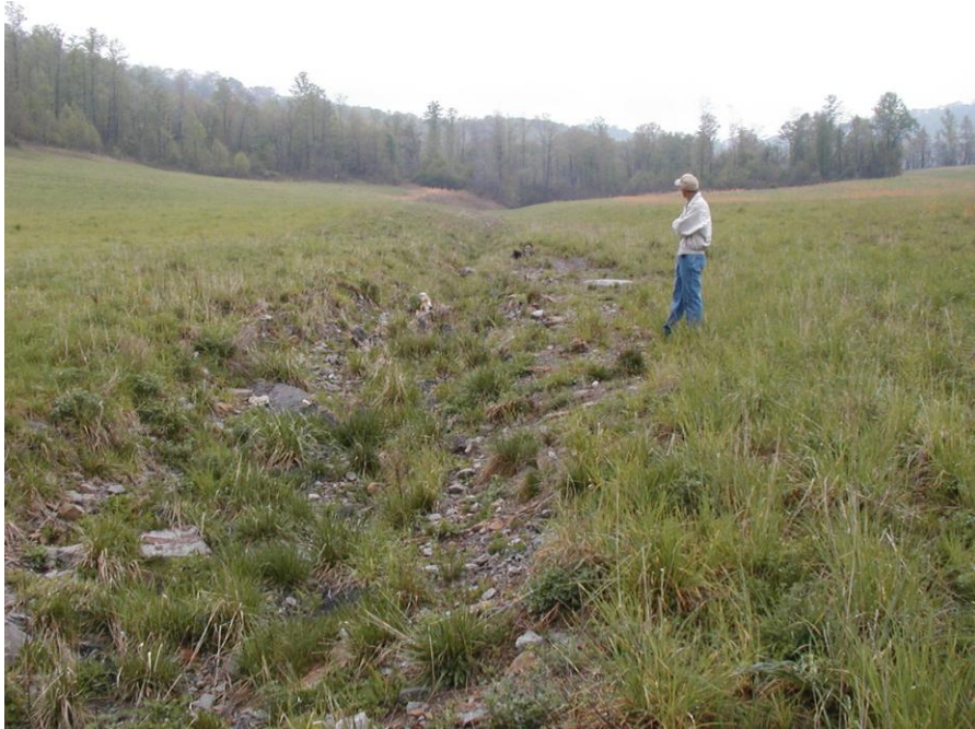
Figure 13. Constructed channel at site1008-95 appears correctly sized for bankfull flow. Flow was directed toward the camera. Imbricated cobbles and pebbles show that this reach has experienced sediment transport although erosion is minimal. J.S. Kite photo.
