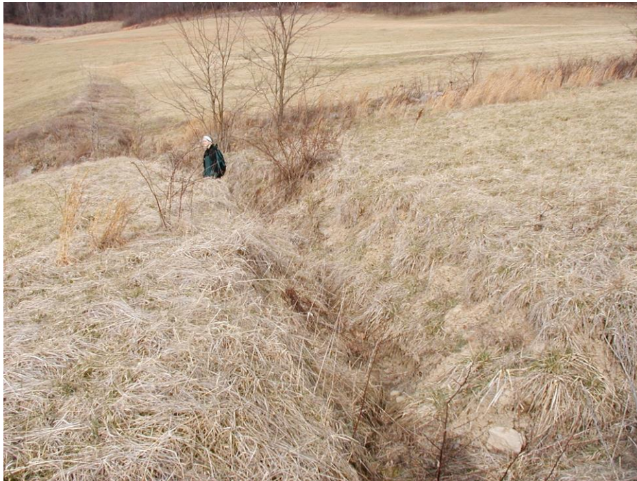
Figure 10. Bermed channel on a south-facing slope at study site 80-80. Channels have been incised by knick-point erosion. J.S. Kite photo.
