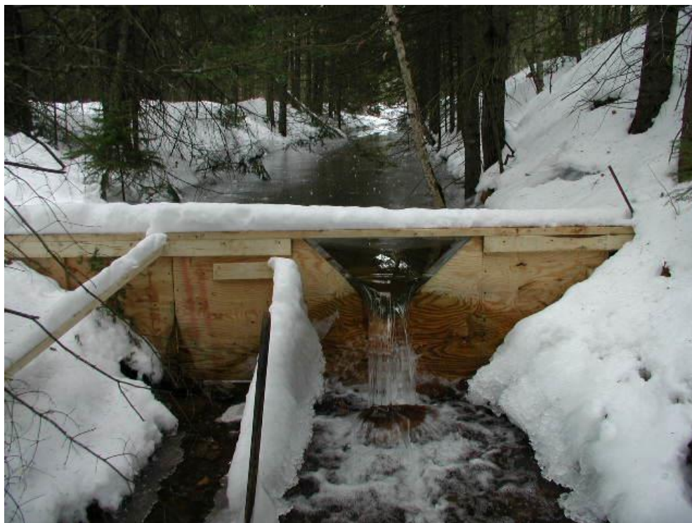
Figure 3. The 90° v-notch weir near the mouth of Ely Brook, Vershire, VT, prior to spring runoff in 2002.
