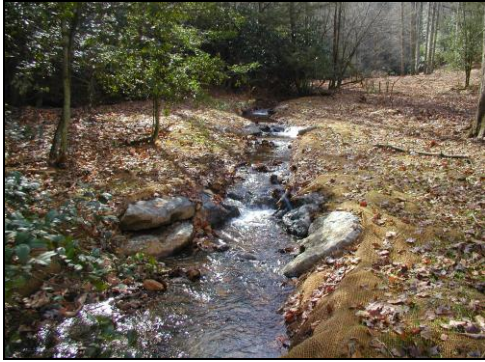
Figure 6. Constructed step/pool channel
