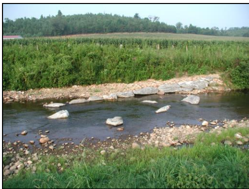
Figure 4. J-hook vane with boulder cluster
