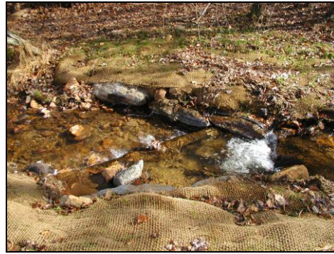
Figure 7. Cross vane with log double drop.
