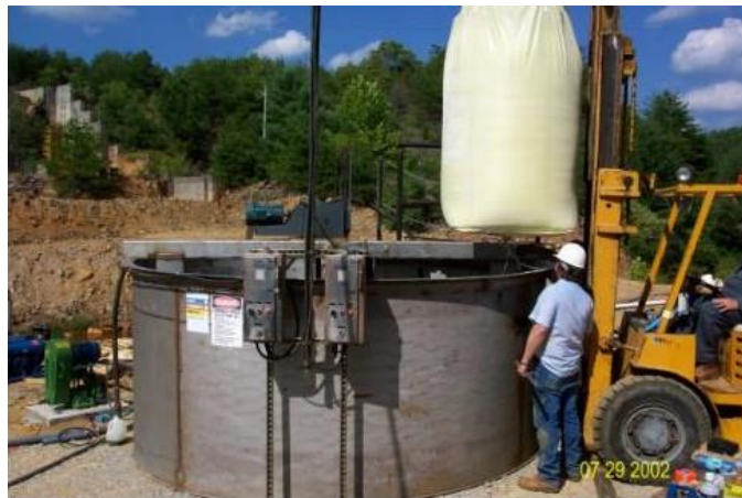
Figure 4. Lime mixing tank
