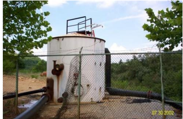
Figure 3. Rapid mix tank
