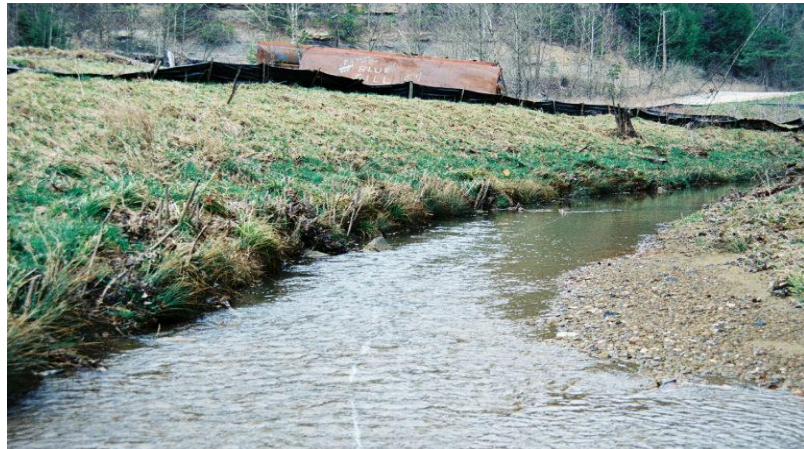
Figure 4: View of Reference Reach
