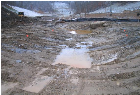
Figure 5. View of Lynn Bark After Excavation
