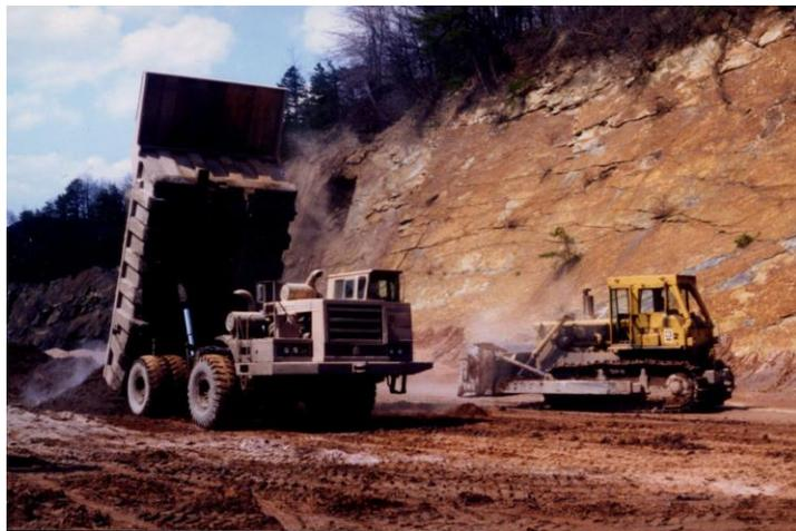
Figure 4. Truck and bulldozer placing ash from the lower platform into the Big Gorilla surface mine pool.
