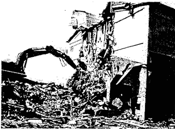
Figure 5 - Demolition of the Breaker Building
