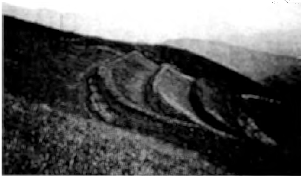
Figure 2. Terraced reclamation hillslope.
