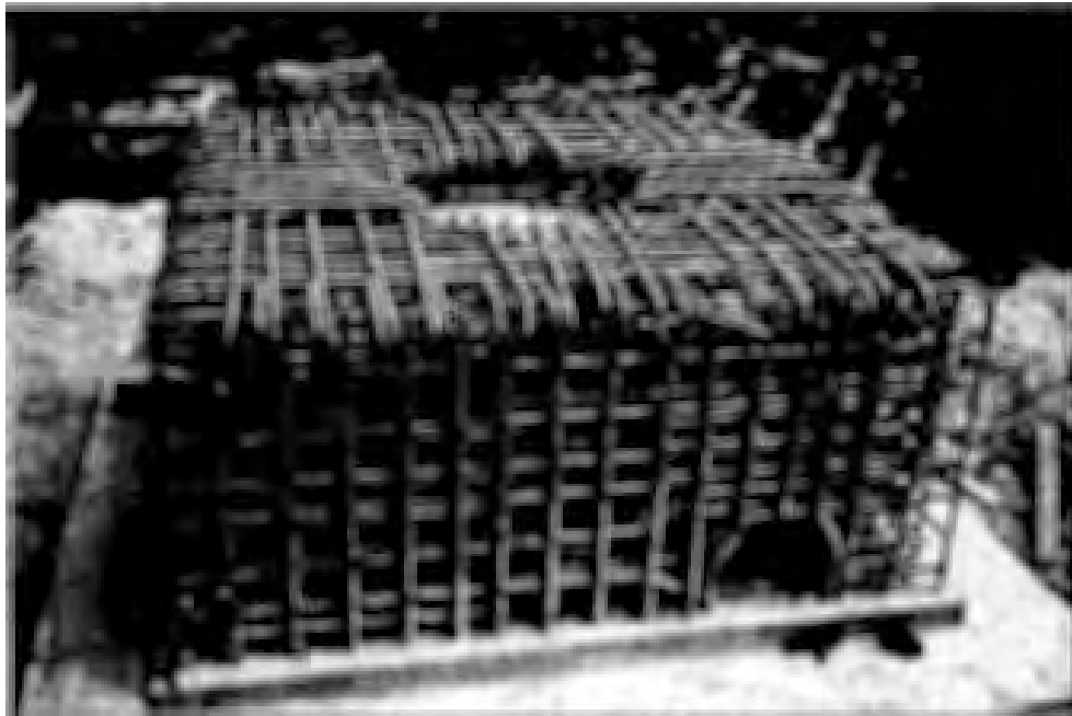
Figure 8. Concrete sump footer and epoxy coated reinforcement steel
