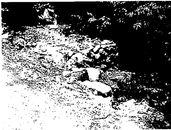
Figure 4 – Check Dam Completely Filled with Sediment
