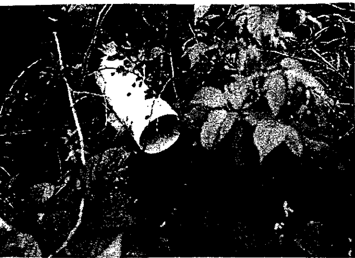
Figure 2(c). 1994 photo of drain on the treated side.
