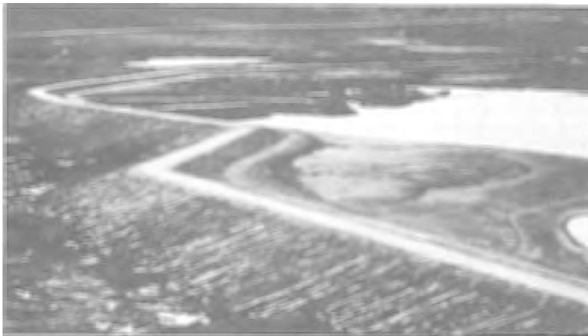
Figure 6. The completed downstream dike.
