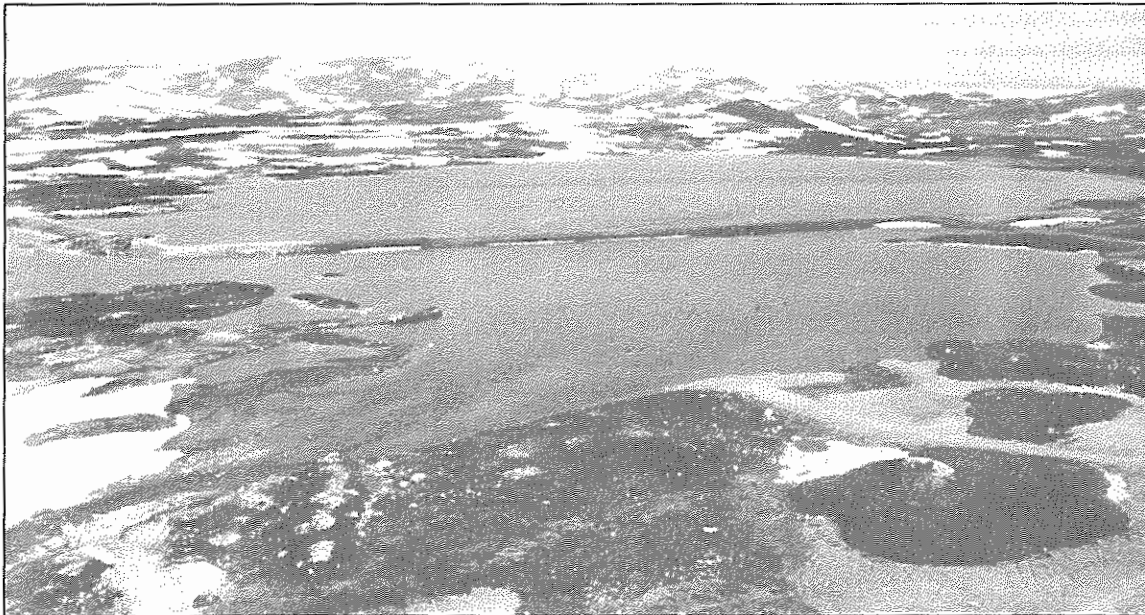
Figure 8. The tailings pond following flooding (the photo's middle and background). Shown in the foreground is the raw water pond.
