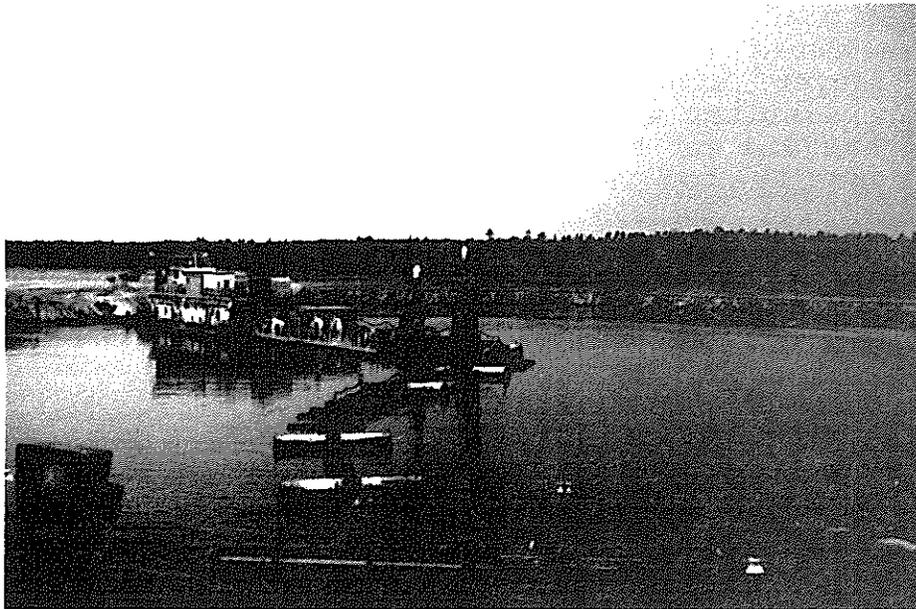
**Figure 1.** Mining dredge at Associated Mineral's mine in Florida. The original topsoil has been removed from the site and the dredge processes the entire subsoil plus mineralized sands to the depth of 10 m. Sandy tailings are deposited behind the dredge and form the subsoil of the new mine soils.
