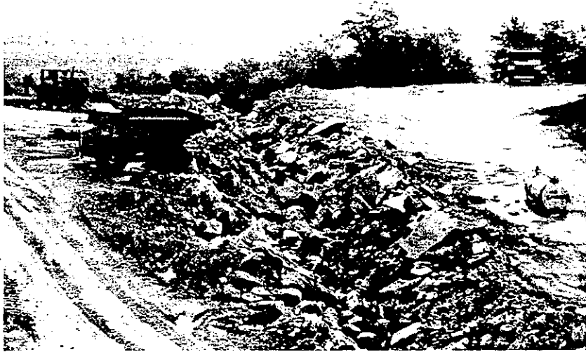
Figure 6. Upper surface of HF2 during the final stage of fill construction, prior to reclamation.
