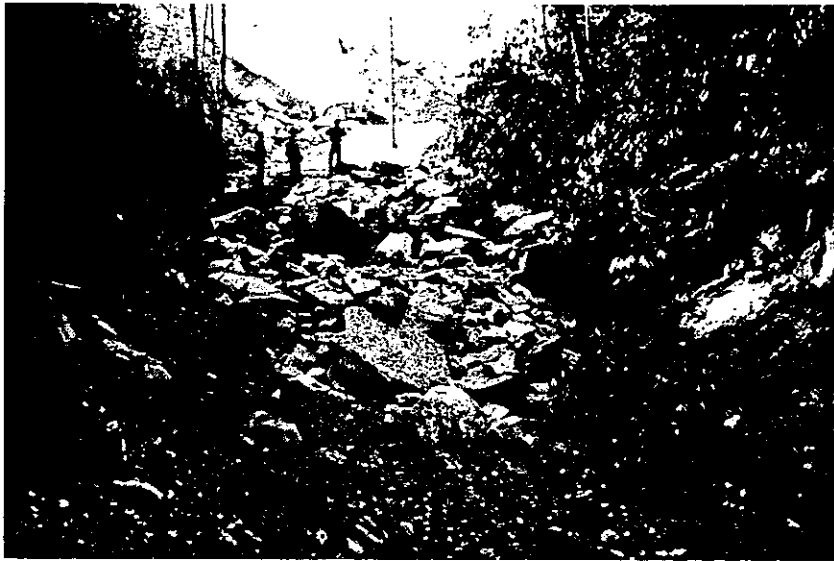
Figure 5. Underdrain of HF3 during construction in December, 1986.
